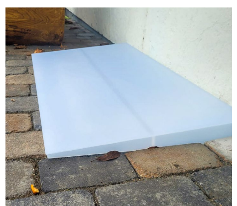
Cellar shaft cover
